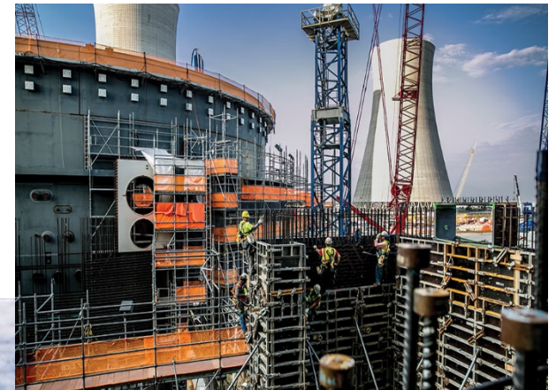
Vogtle Unit 3 Courtesy of Georgia Power
